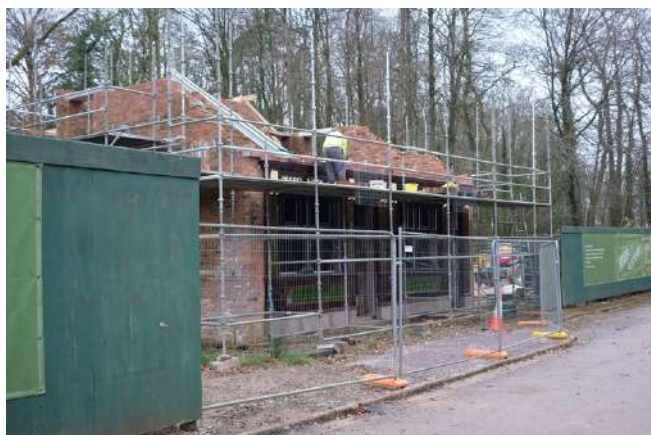
Figure 13 The Vulcan pub reconstruction underway
